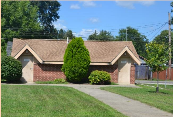
ADA Restrooms with paved sidewalks (facing north)
