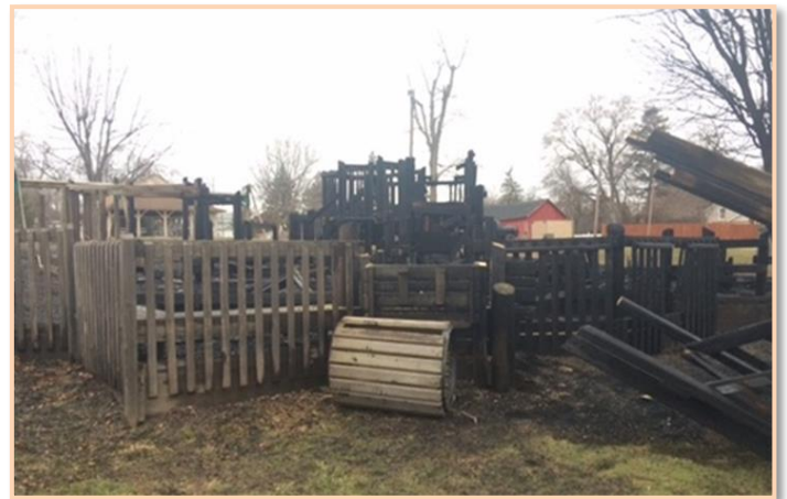
Photo of Fire Damage: Permission to reproduce, WANE 15 (4-2015)
