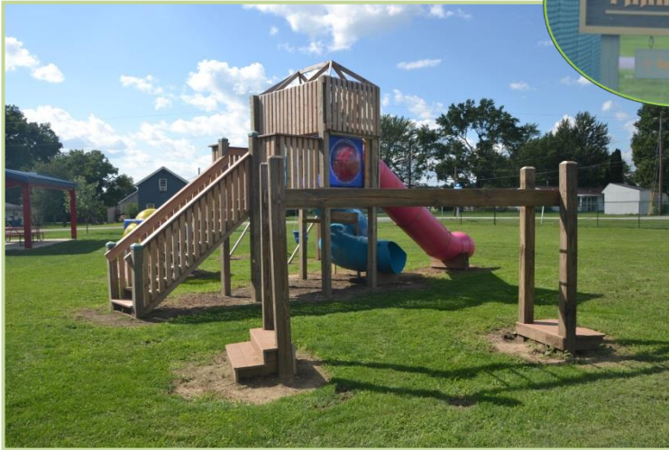
New hanging ladder and play structures (facing southwest)
