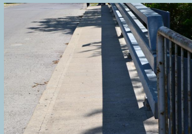
Grade C – Major Deficiency: For instance, the sidewalk shown here is too narrow and has joint displacements making it complicated to navigate by wheelchair, though still passable for someone walking.
