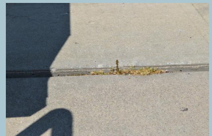
Grade C – Major Deficiency: For instance, the sidewalk shown here is too narrow and has joint displacements making it complicated to navigate by wheelchair, though still passable for someone walking.
