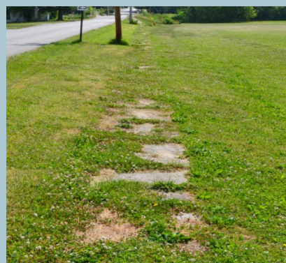
Grade D - Multiple Major Deficiencies: For instance, the sidewalks shown here are too narrow, they have joint displacements, rough/cracked surfaces, and gaps making it likely impassable by wheelchair, though a fit walker could still navigate the sidewalk.
