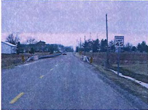
Figure 8: Looking north along Minnich Road
