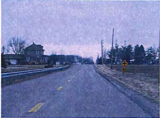
Figure 9: Looking north along Minnich Road
