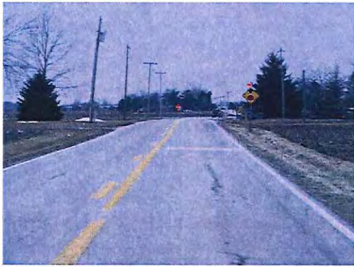
Figure 1: Looking west along Tillman Road
