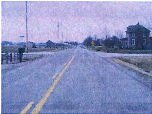
Figure 14: Looking south along Minnich Road
