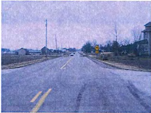
Figure 15: Looking south along Minnich Road
