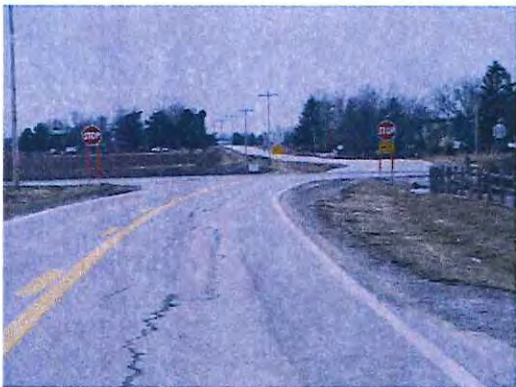
Figure 3: Looking west along Tillman Road
