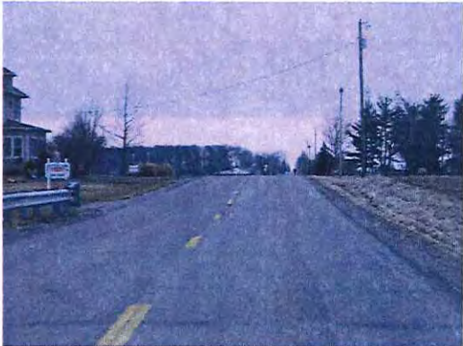
Figure 10: Looking north along Minnich Road
