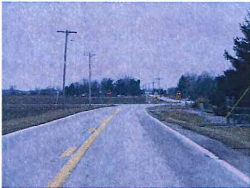
Figure 2: Looking west along Tillman Road
