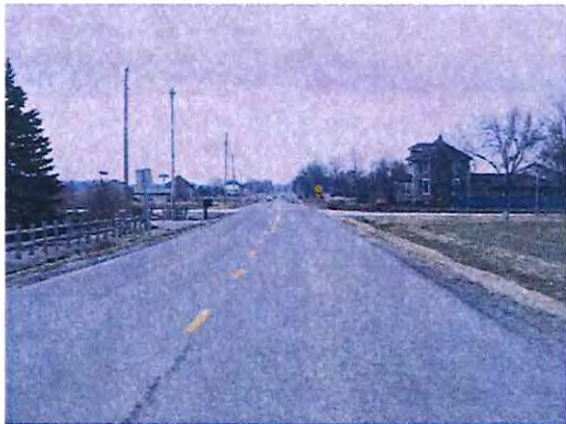
Figure 13: Looking south along Minnich Road
