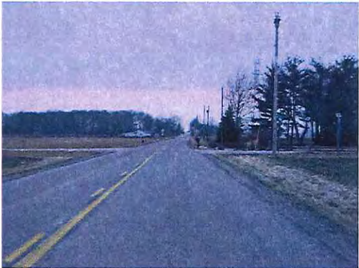
Figure 11: Looking north along Minnich Road
