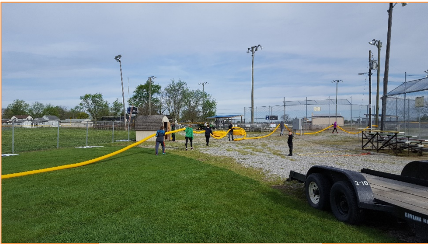
New safety fencing covers
