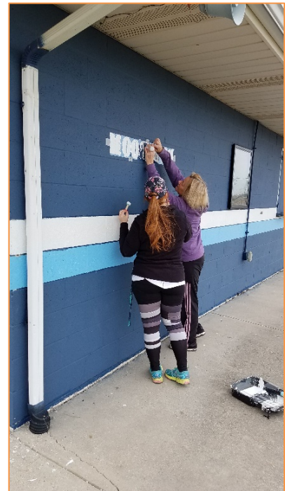
Restroom paint improvements
