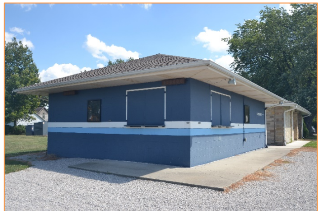
2-Bay Concession Stand / Restrooms (facing southeast)
