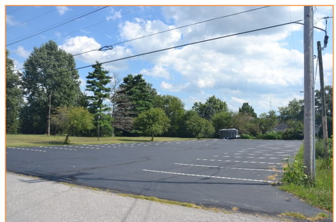
Asphalt parking area (facing southeast)
