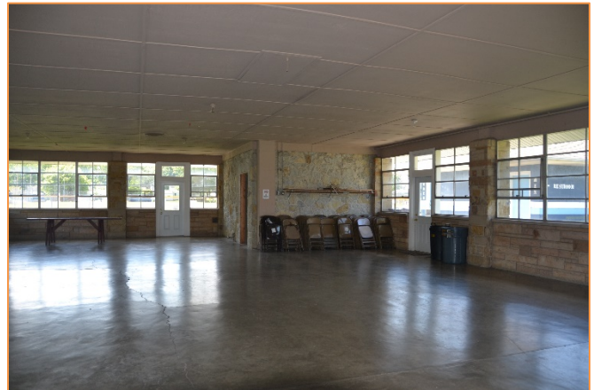
Inside Shelter House (facing west at exit areas)
