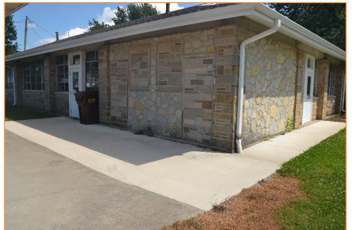
New gutters and soffit at Shelter House
