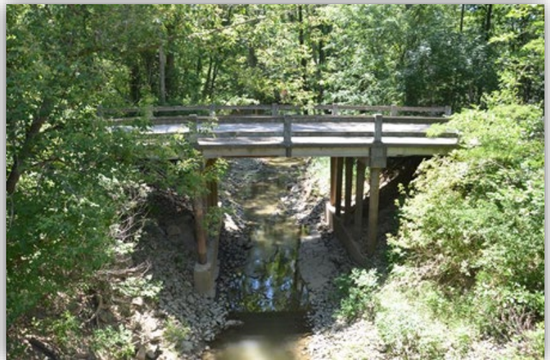
Outstanding Historic Bridge, Source: DNR-DHPA, SHAARD website (photo downloaded 11-27-19)
