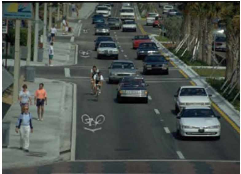
Examples of a Wide Curb Lane
