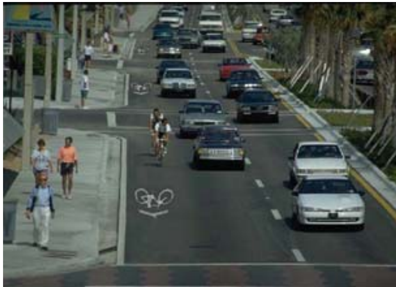
Examples of a Wide Curb Lane
