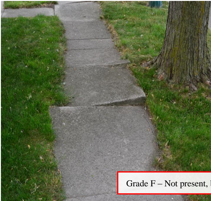
Grade D – Multiple Major Deficiencies: For instance, the sidewalks shown here are too narrow, they have joint displacements, rough/cracked surfaces, and gaps making it likely impassable by wheelchair, though a fit walker could still navigate the sidewalk.
