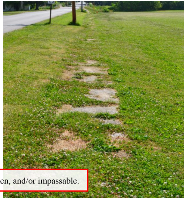
Grade D – Multiple Major Deficiencies: For instance, the sidewalks shown here are too narrow, they have joint displacements, rough/cracked surfaces, and gaps making it likely impassable by wheelchair, though a fit walker could still navigate the sidewalk.
