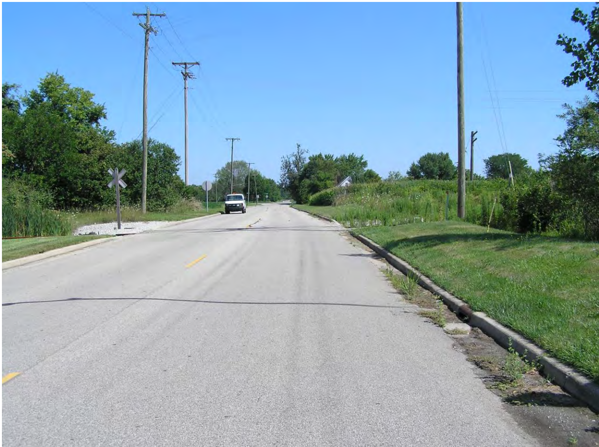
Industrial Park Drive (northbound)
