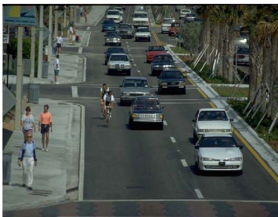
Example of a Wide Curb Lane
